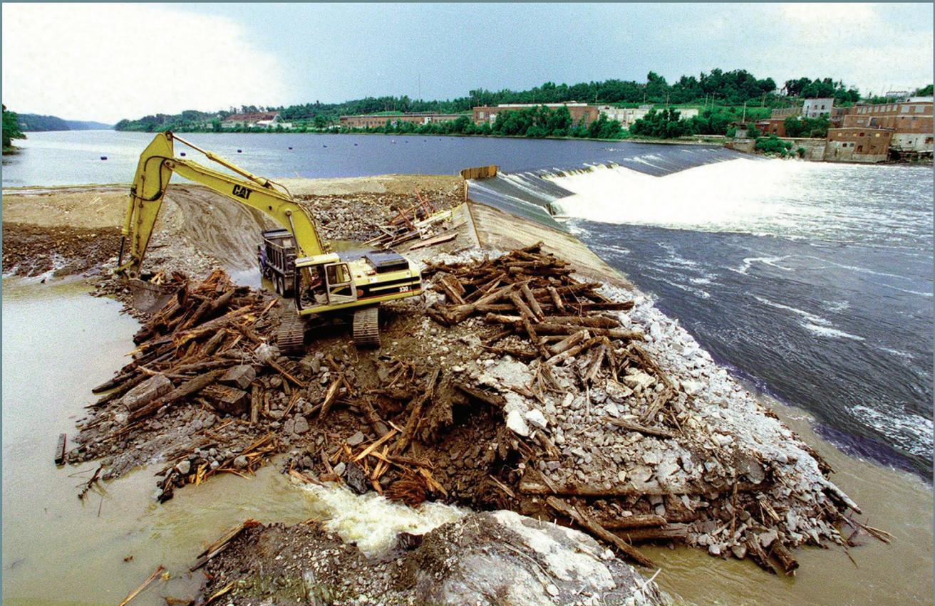
A backhoe begins work June 24, 1999, on removing the 850-foot-long Edwards Dam in Augusta, Maine, built in 1837 and constructed of a cribwork of logs and stone and later capped with concrete. When the dam is breached the water level will drop 10 feet behind the dam. Photo Credit: Kennebec Journal
